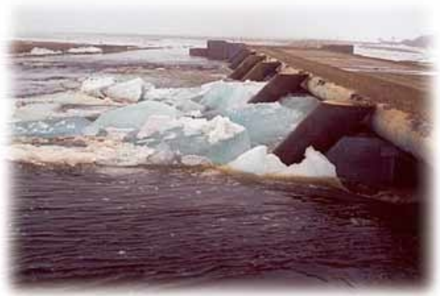
Figure 3. Five-ft (1.5 m) thick fresh water ice impacting the bridge. The thin superstructure with rounded upstream nose and the sloped ice breaking pipes were all designed to minimize the ice loading on the submersible bridge, and to provide ice passage over or under the bridge.
