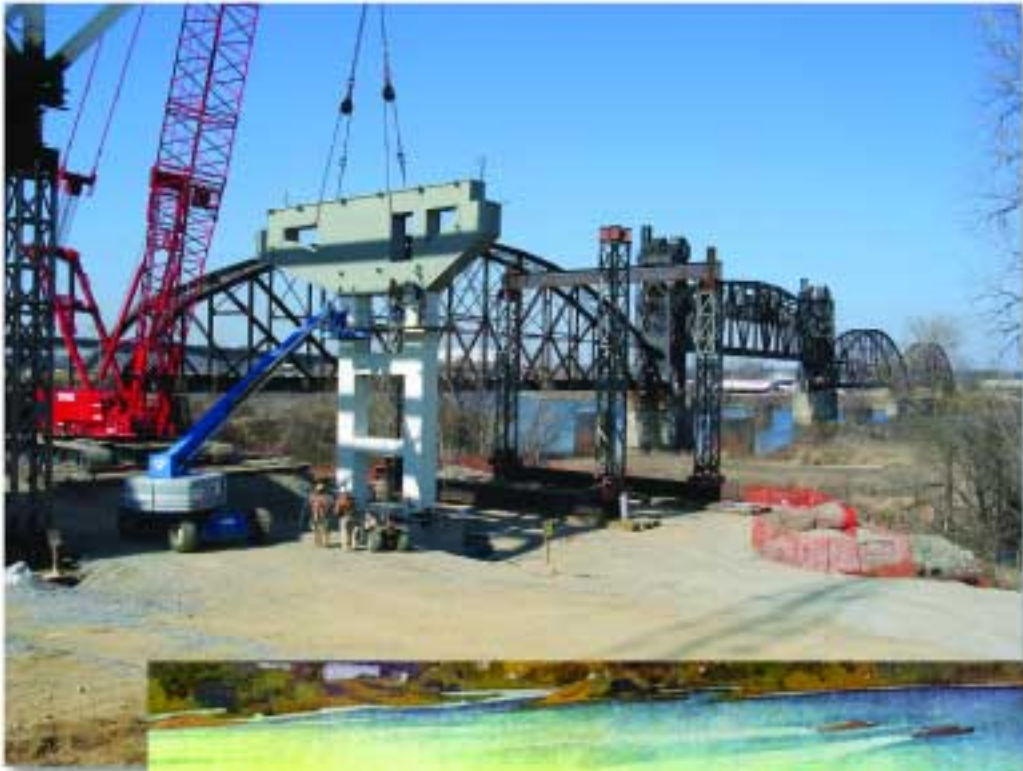
Figure 4. ◀ Cap girder erection on pier.
