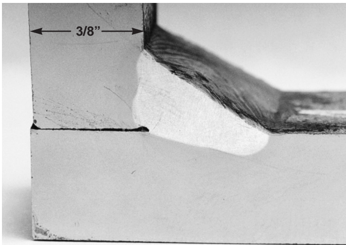
Figure 4. The use of SAW does not guarantee penetration beyond the root.
