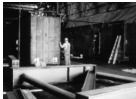
Figure 3. Fabrication of the 6 by 10 ft (1,800 mm by 3,000 mm) box beam sections.
