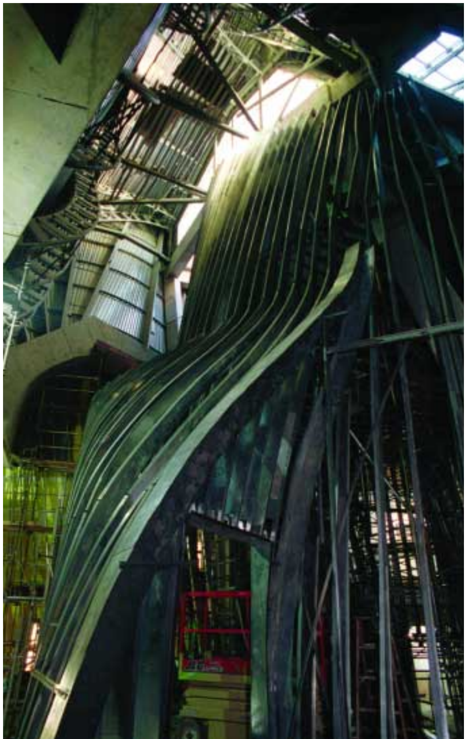
This soaring structural steel framework is now hidden by the outer skin and inner walls of the building.
