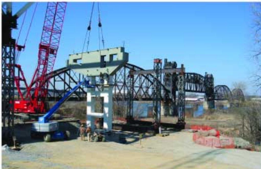
Figure 4. Cap girder erection on pier.
