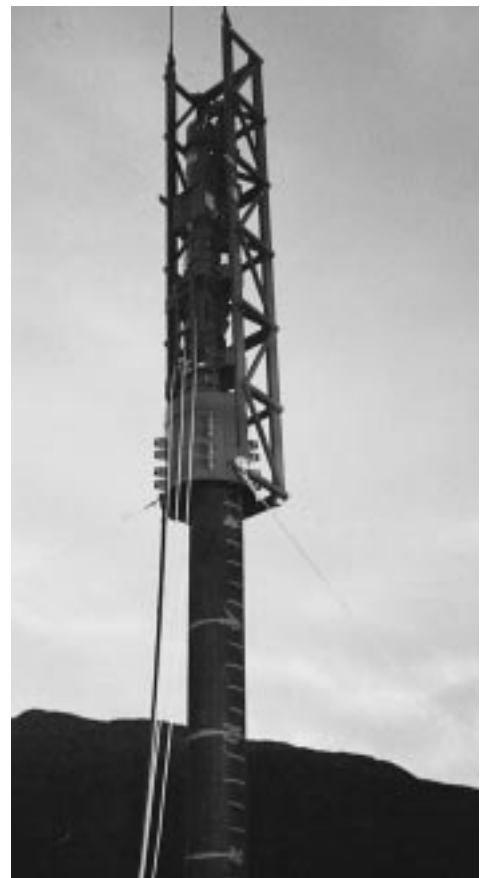
Figure 3. Driving the anchor pile with a diesel impact hammer.
