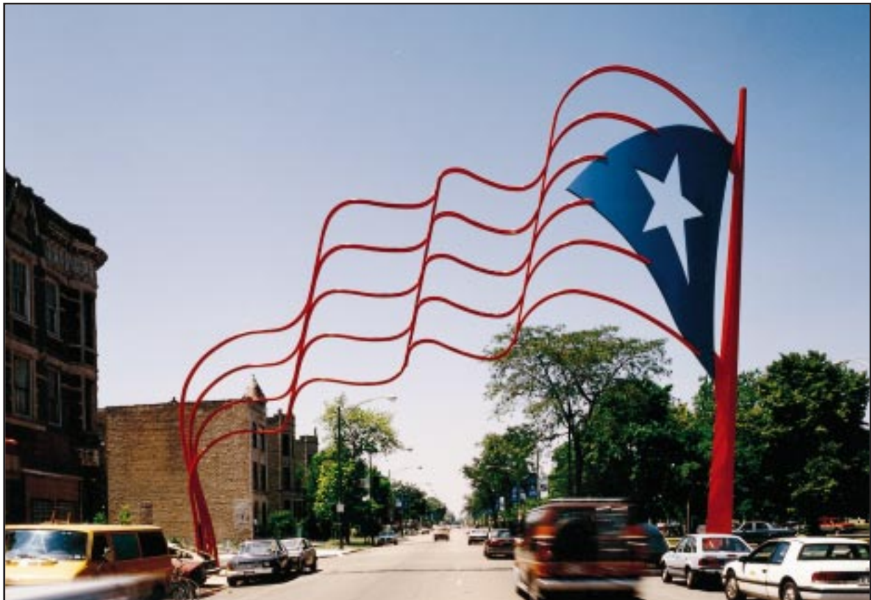
This all-welded sculpture of the Puerto Rican flag is one of two “gateway” structures designed for a community commercial district. See story on page 23.
