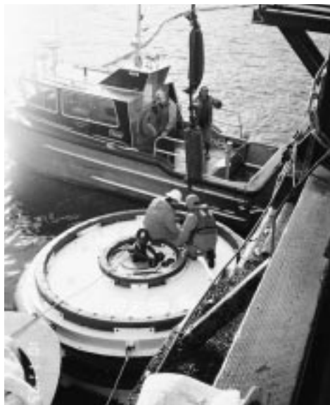
Figure 4. Final connection of the mooring buoy to the mooring chain.
