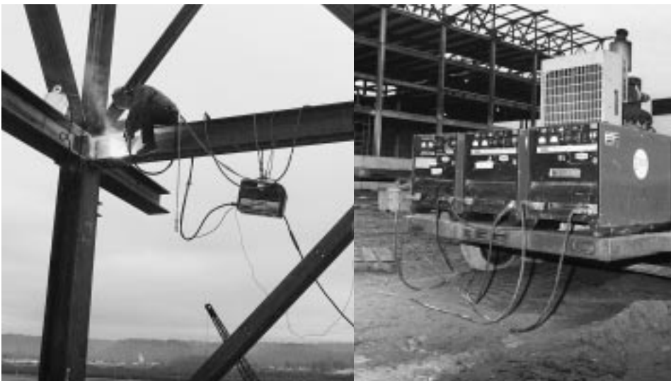
Figure 2. The arc voltage is always lower than the machine voltage due to the resistance of the welding cables.
