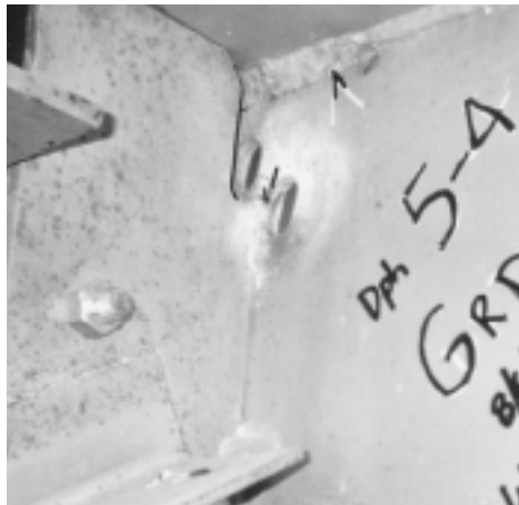
(b) south side of connection plate
