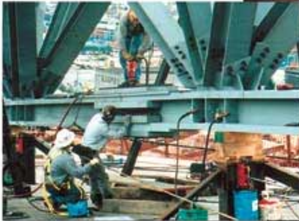
Figure 4. Erection crew assembling truss.
