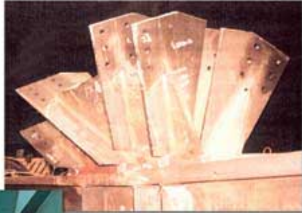
Figure 3. Bottom chord assembly at the splice location with welded diagonal connections.
