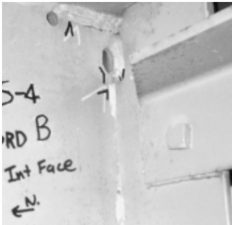
(a) north side of connection plate
