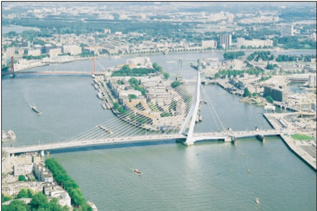
Fondly referred to by city residents as “The Swan,” the Erasmus Bridge enhances both the skyline and traffic flow in Rotterdam, the Netherlands. The welded, cable-stayed structure was fabricated using Lincoln Smitweld products. Story on page 19.
