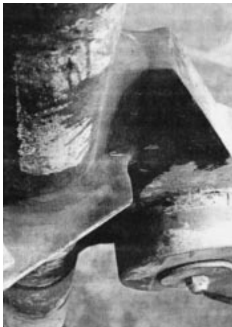
Figure 7. Weld joints ground smooth to enhance resistance to fatigue.
