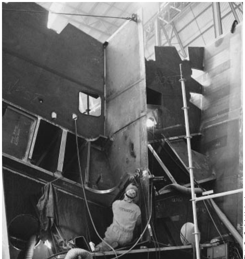
Figure 4. A section of the pylon being fabricated using Lincoln Smitweld products.
