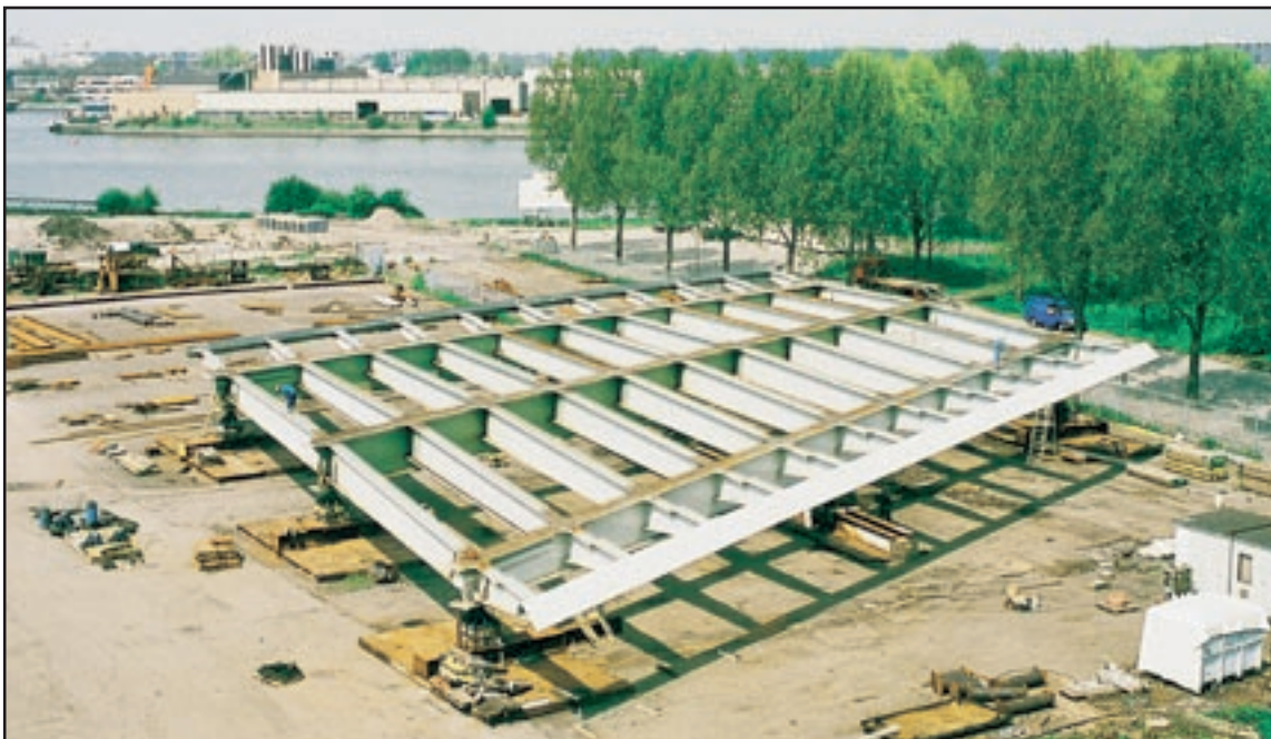
Figure 8. The complete steel construction of the bridge during building.
