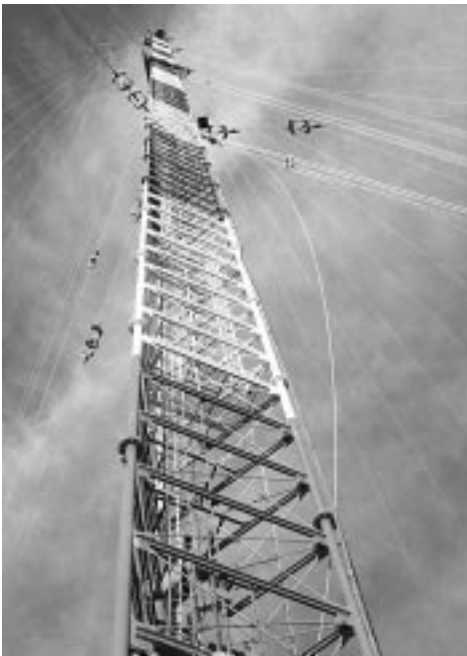
Figure 6. Weld repairs were successfully made to this 1,200 ft (365 m) radio tower.
