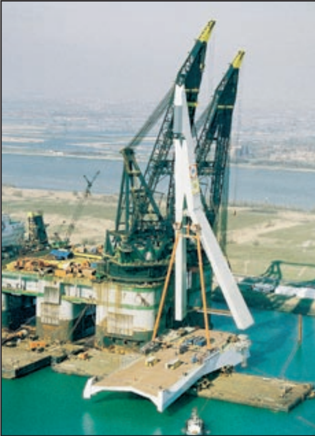
Figure 6. An offshore craneship puts the pylon on the back span.
