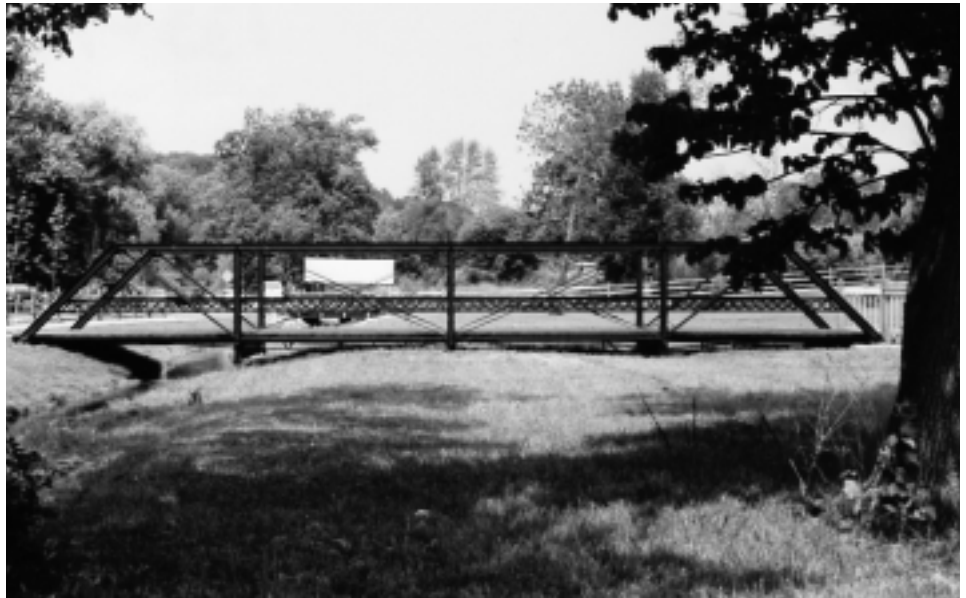
Figure 1. The rehabilitated 133rd Avenue bridge, installed at the Calhoun County Historic Bridge Park.
