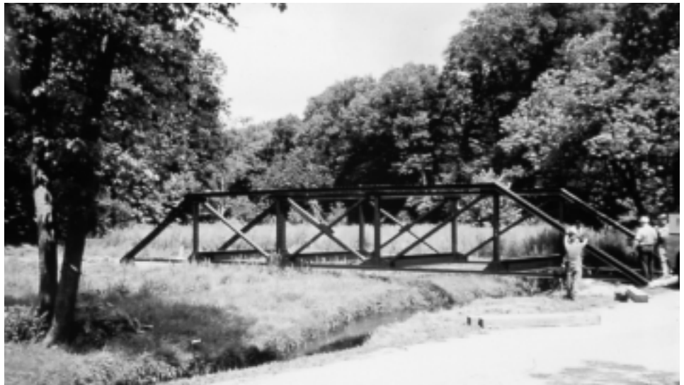
Figure 2. The rehabilitated Twenty Mile Road bridge, shown in its new position at the Historic Bridge Park.
