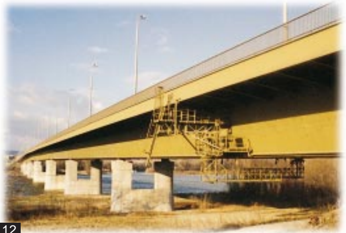
Figure 10. The cable stayed bridge over the Danube at Novi Sad, Yugoslavia, 1981 (spans: 4x60.0 + 2x60.0 + 351.0 + 2x60.0 + 3x60.0 m).
