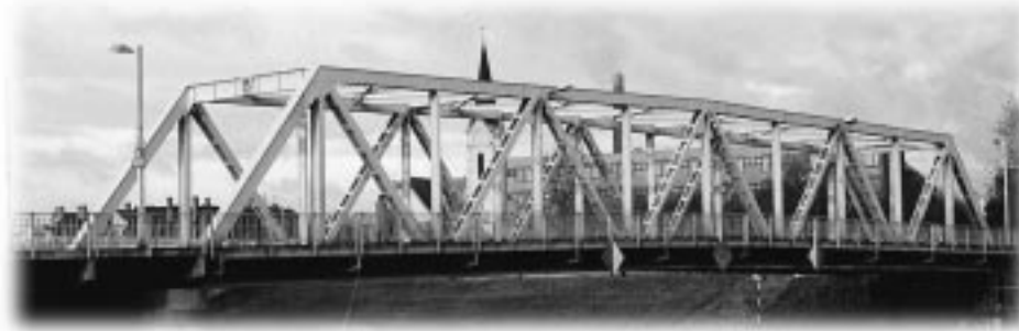
Figure 1. The first welded bridge in Hungary, at Győr, opened in 1935 (span: 53.1 m).
