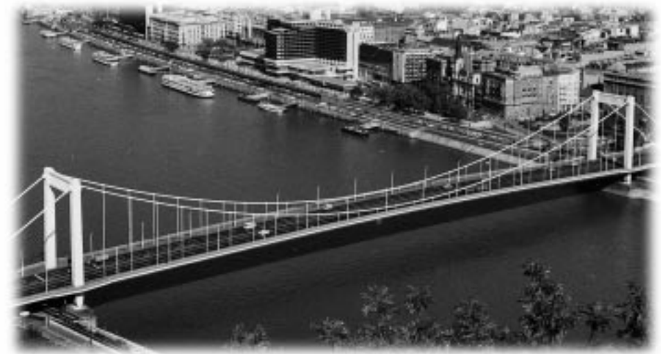
Figure 5. The Erzsébet cable bridge at Budapest, shown today (spans: 44.3 + 290.0 + 44.3 m).
