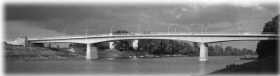
Figure 2. The first bridge in Hungary with a fully welded orthotropic deck spans the Tisza River at Szolnok, and was opened in 1962 (spans: 54.8 + 79.3 + 54.8 m).
