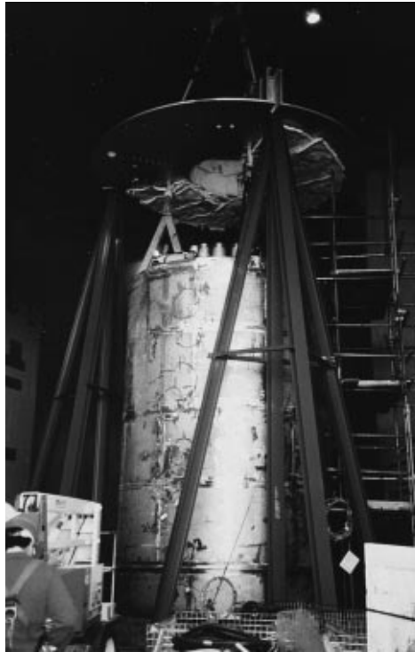
The heat exchanger prior to its installation inside the reactor vessel.
