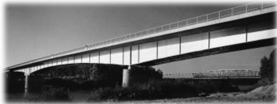
Figure 6. The composite bridge over the Tisza at Algyó has spans of 57.6 + 102.4 + 57.6 m.
